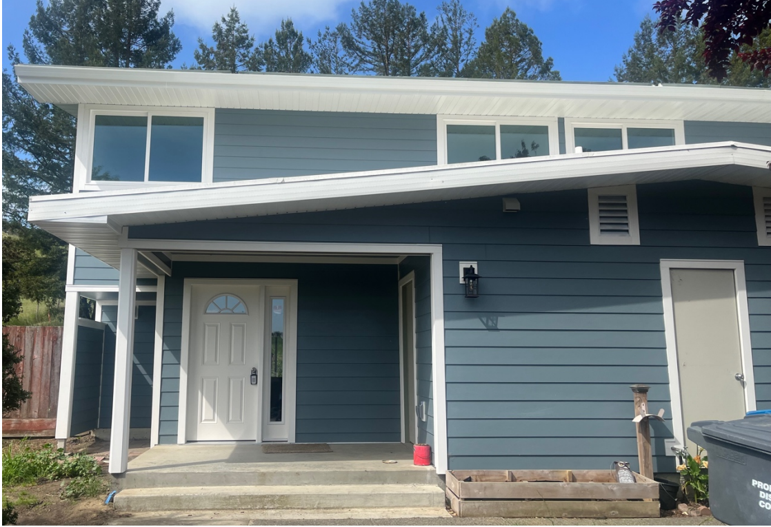
FRONT OF THE HOME
