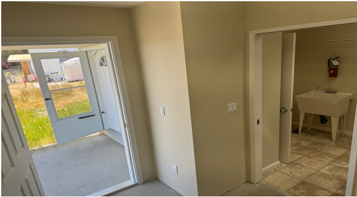
Entrance Storage room view
