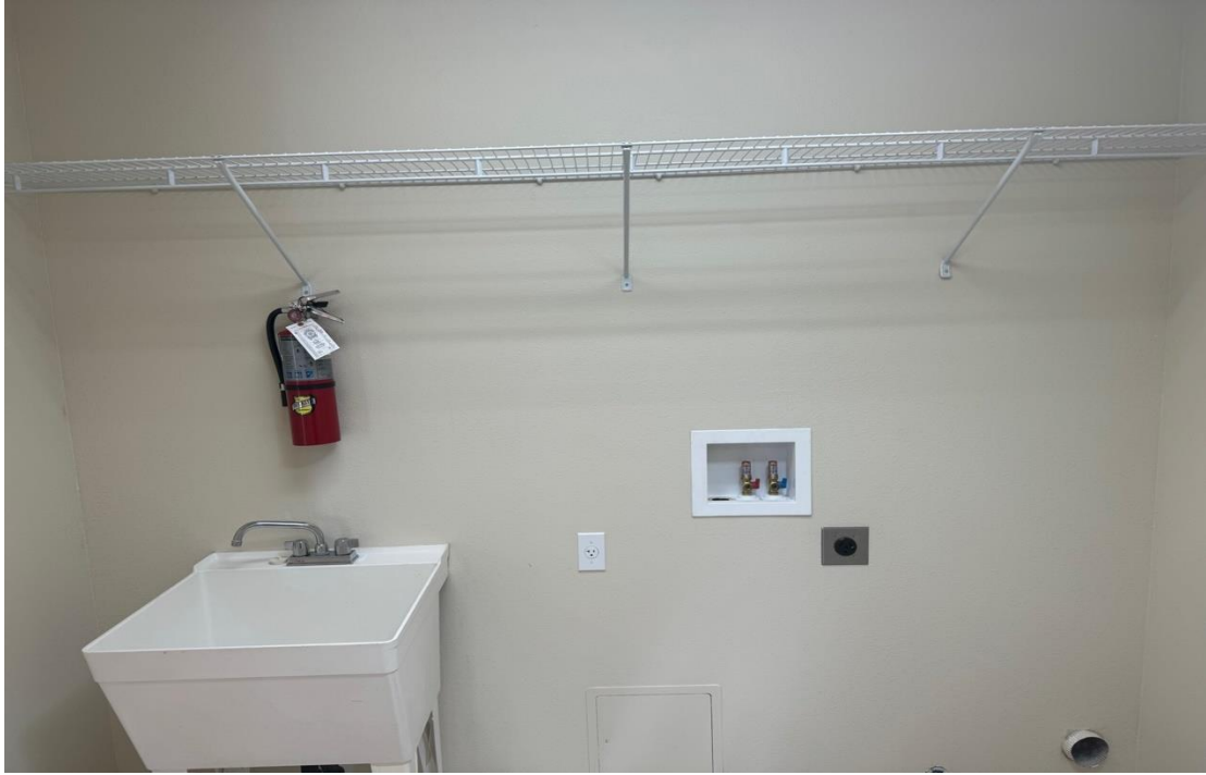
Laundry room View (Gas does not work) Electrical only
